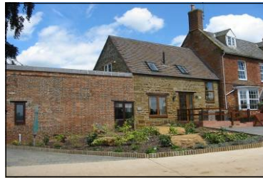
The Granary was built using local Northamptonshire stone with walls 2 feet thick!
